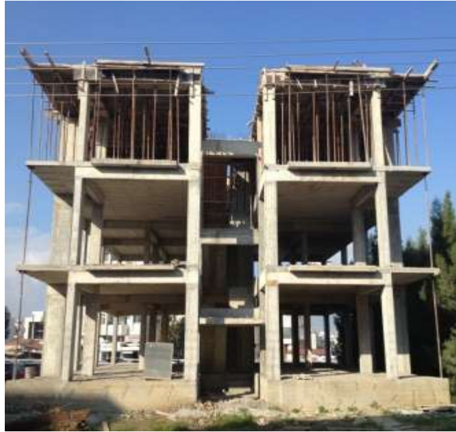
Picture 1. Rough construction of an ordinary apartment building in Nicosia.
